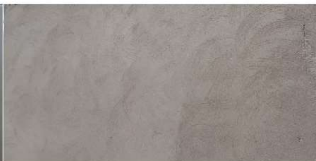
Rough Cast Plaster Finish
